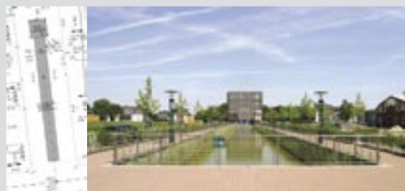
Drainage basins with the Lamellenhaus
