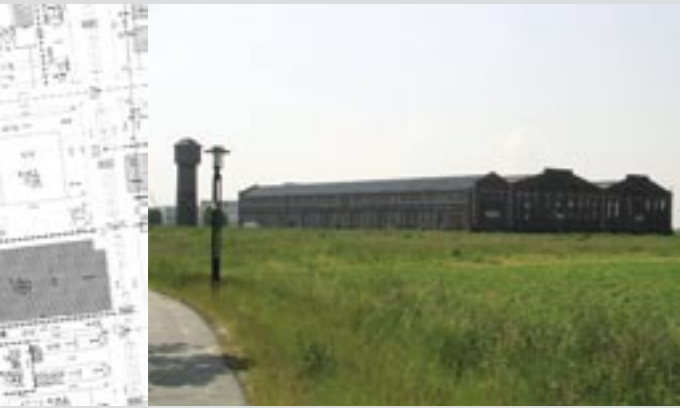
View of Hall 4 from the entrance of the business park
